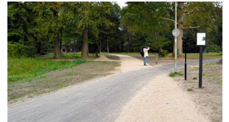
Referentie wandelpaden: halfverhard pad (Twickels padvast)
