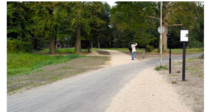
Referentie wandelpaden: halfverhard pad (Twickels padvast)
